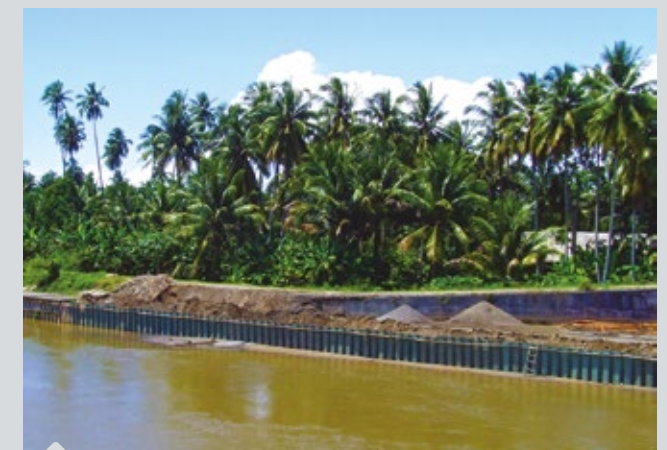
Erosie bescherming in de rivierbedding.
